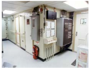
RED LINE PKP Extinguisher Installation.jpg
