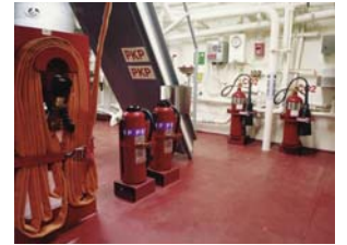
RED LINE PKP- CO2- and Niedner Hose Install.jpg
